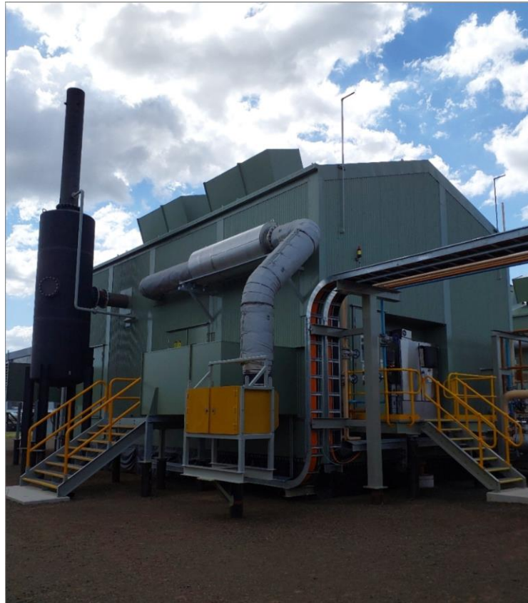
Figure B3: Engine Exhaust Muffler (Maxim) from ACS-03 Site.
