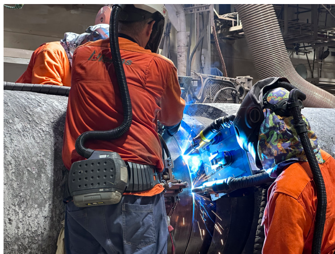
Welding of pipeline sections aboard the Audacia
