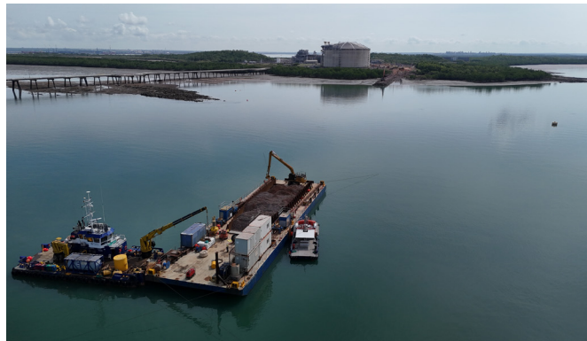
Installation of rock protection over the pipeline at the shore crossing
