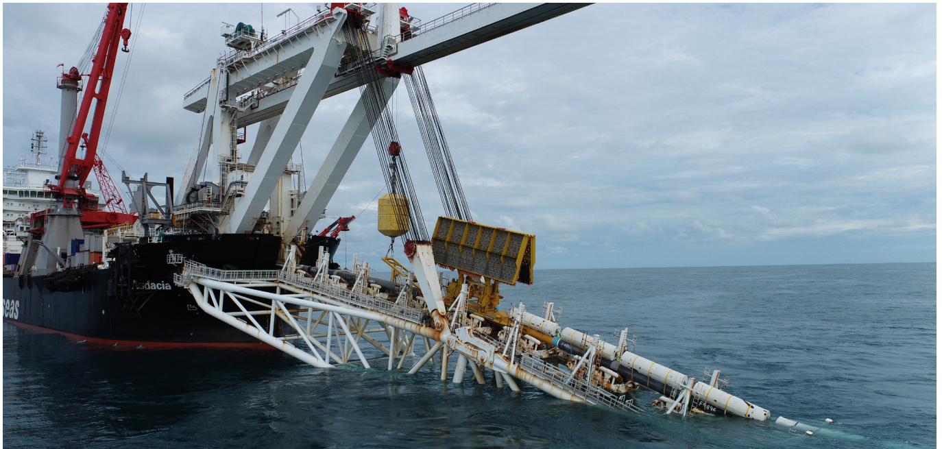
Audacia installing the pipeline.
