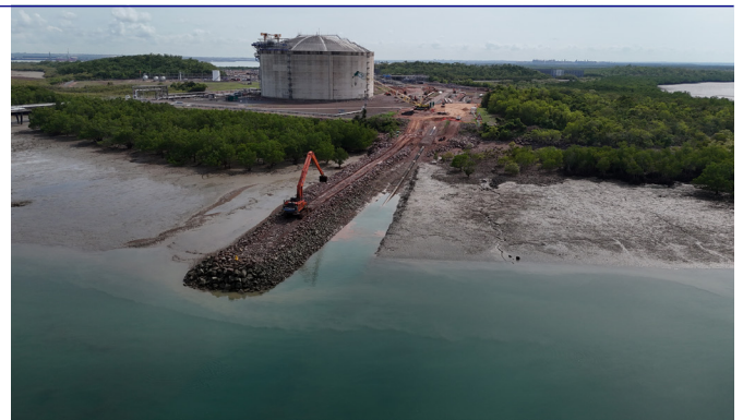
Rock installation at the shorecrossing.
