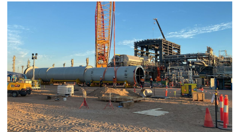
Primary stack positioned for fit up and weld out
