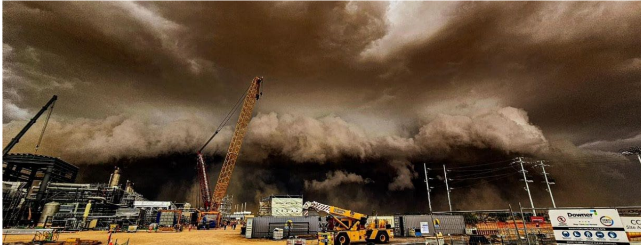
Wet Weather at Moomba CCS phase 1 site in Q1 2024
