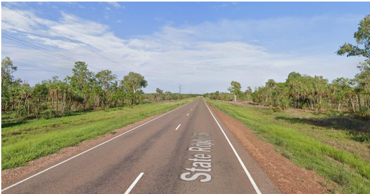
Figure 6-2 Arnhem Highway west of Barr Road, facing east
