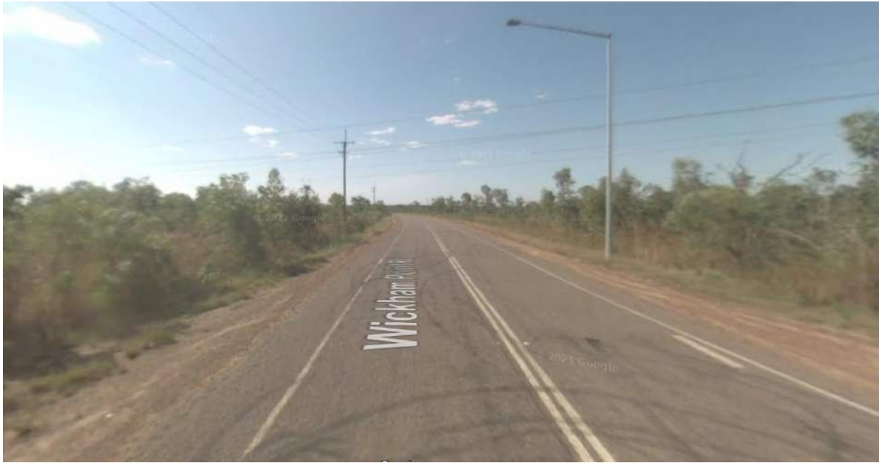
Figure 6-15 Wickham Point Road north of Channel Island Road, facing north
