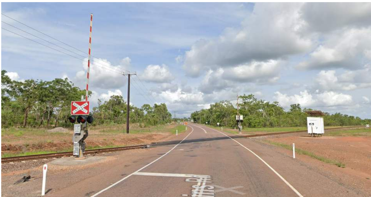
Figure 6-12 At grade level crossing Jenkins Road facing west, 600 m east of Channel Island Road
