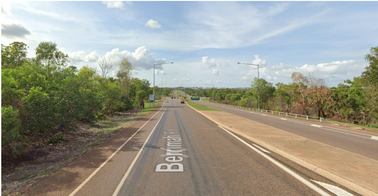
Figure 6-5 Berrimah Road north of Tiger Brennan Road, facing south
