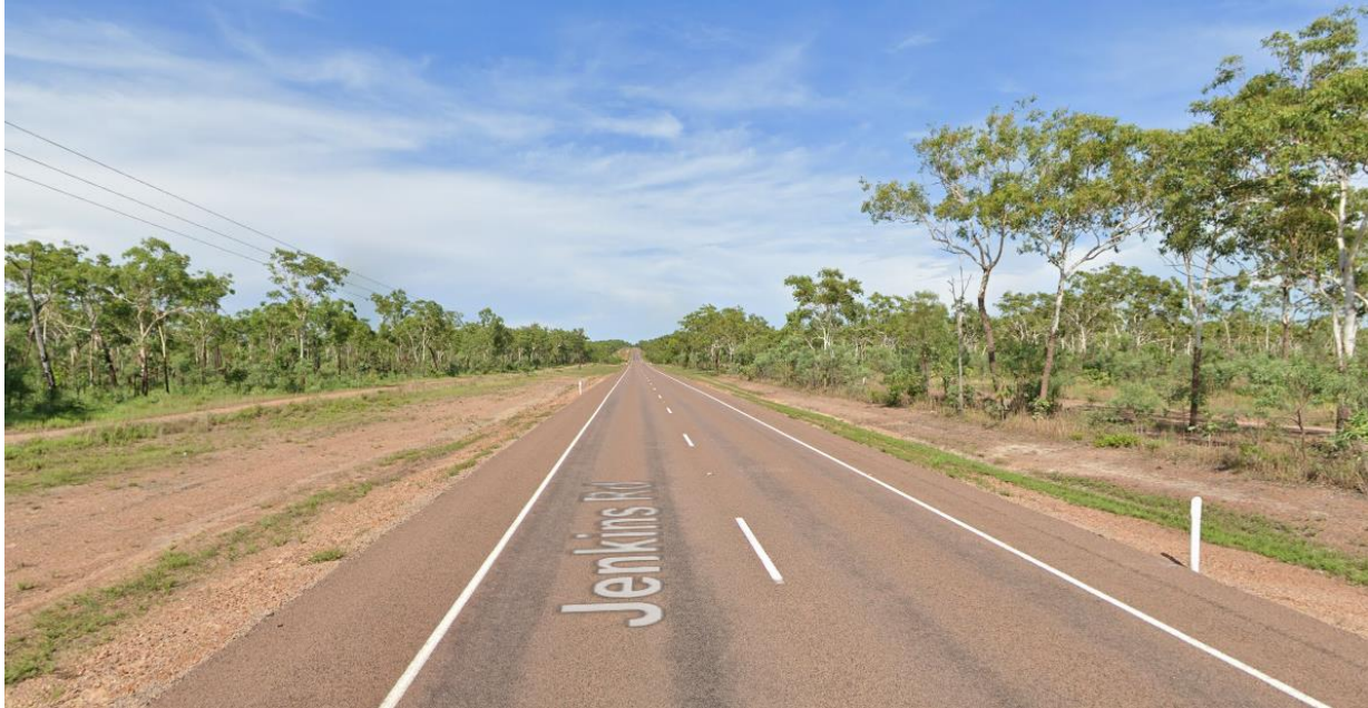
Figure 6-11 Jenkins Road west of the Stuart Highway, facing west
