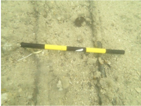
Figure 51: Image of the two parallel lies of communication cable laying on sea floor. (Source: CA 2012).
