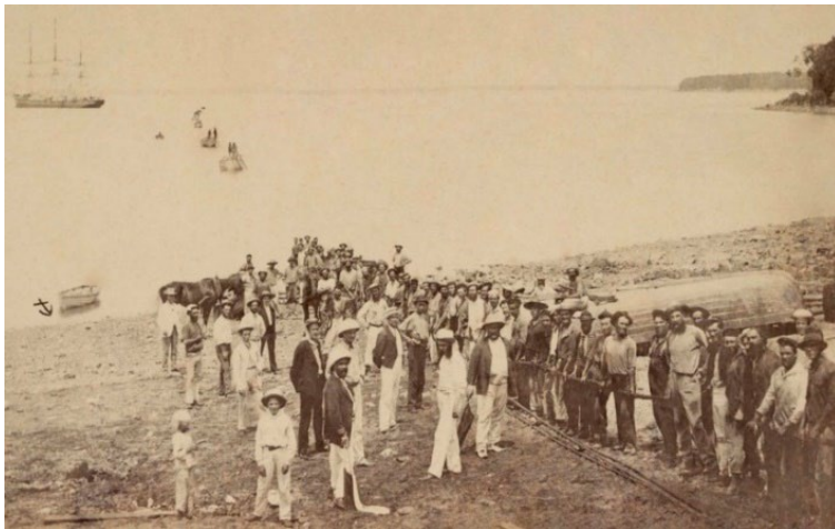
Figure 6: Landing the telegraph cable, Darwin, 1871. 44
