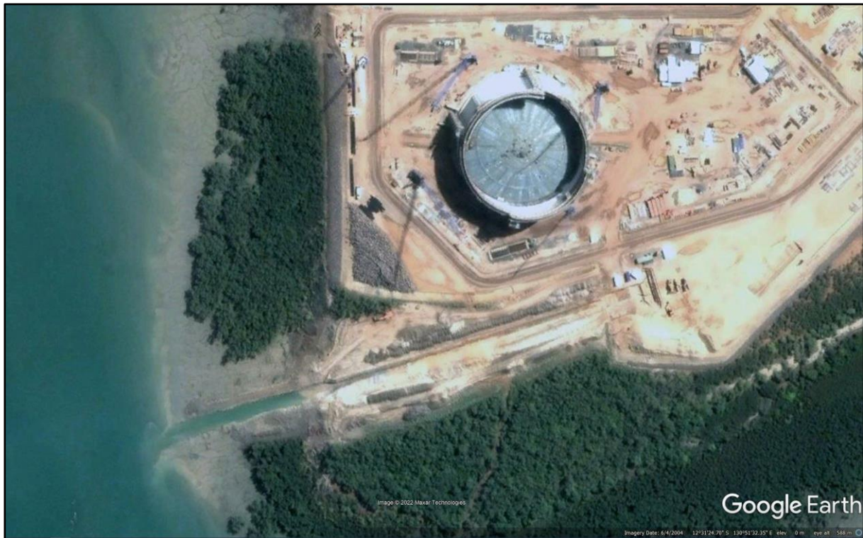
Figure 2-6: Aerial image of the site and surrounds – June 2004 (Image source: Google Earth, accessed: 19/08/22)
