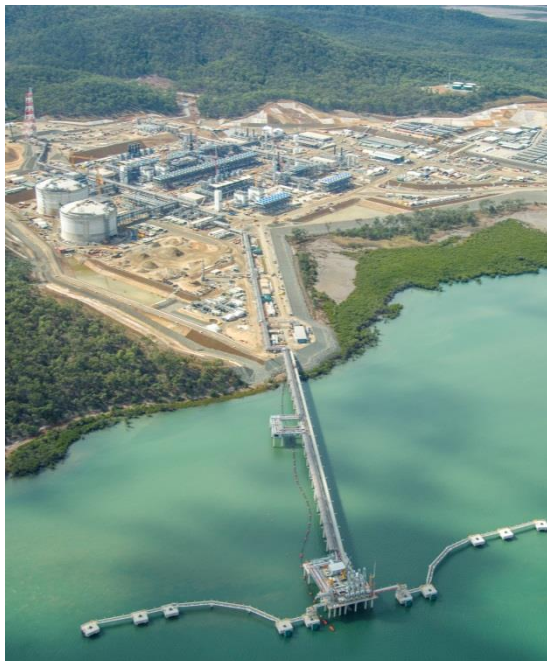
GLNG, Curtis Island, Queensland
