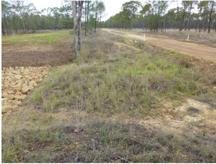
Powerline RoW 45 easement
