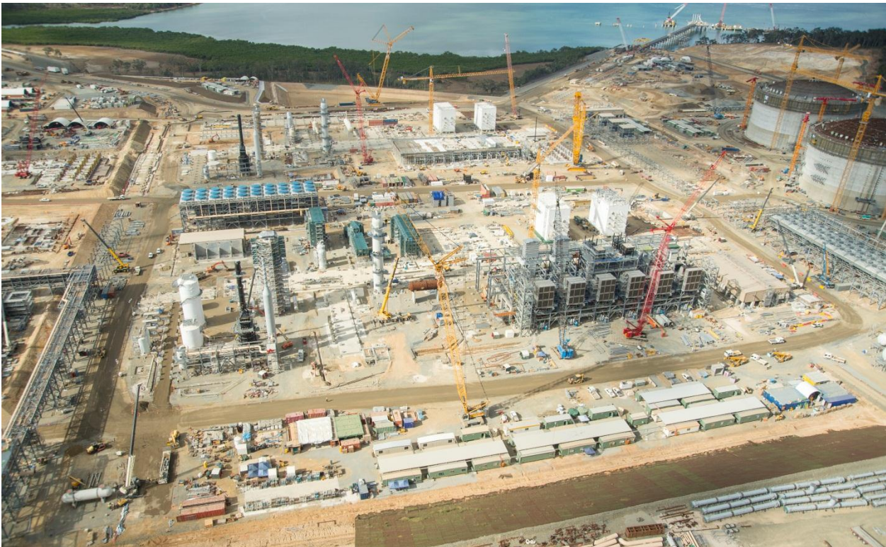
Construction of LNG train 1 (foreground) and train 2 on Curtis Island, September 2013.
