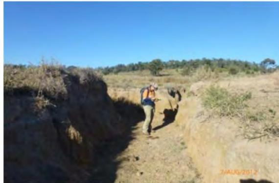
Photo 140 Severe erosion of dam overflow at KP292.45
