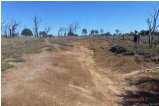
Photo 109 Erosion on existing track at KP266.50
