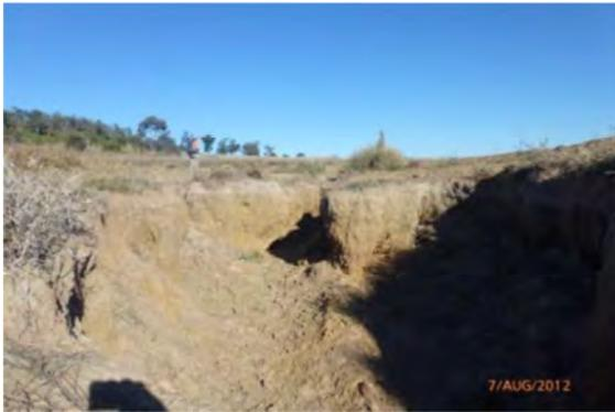
Photo 139 Severe erosion of dam overflow at KP292.45
