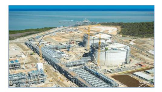
On Curtis Island, as you can see in the photo, the two LNG tanks are progressing well with hydrostatic testing to commence soon.
