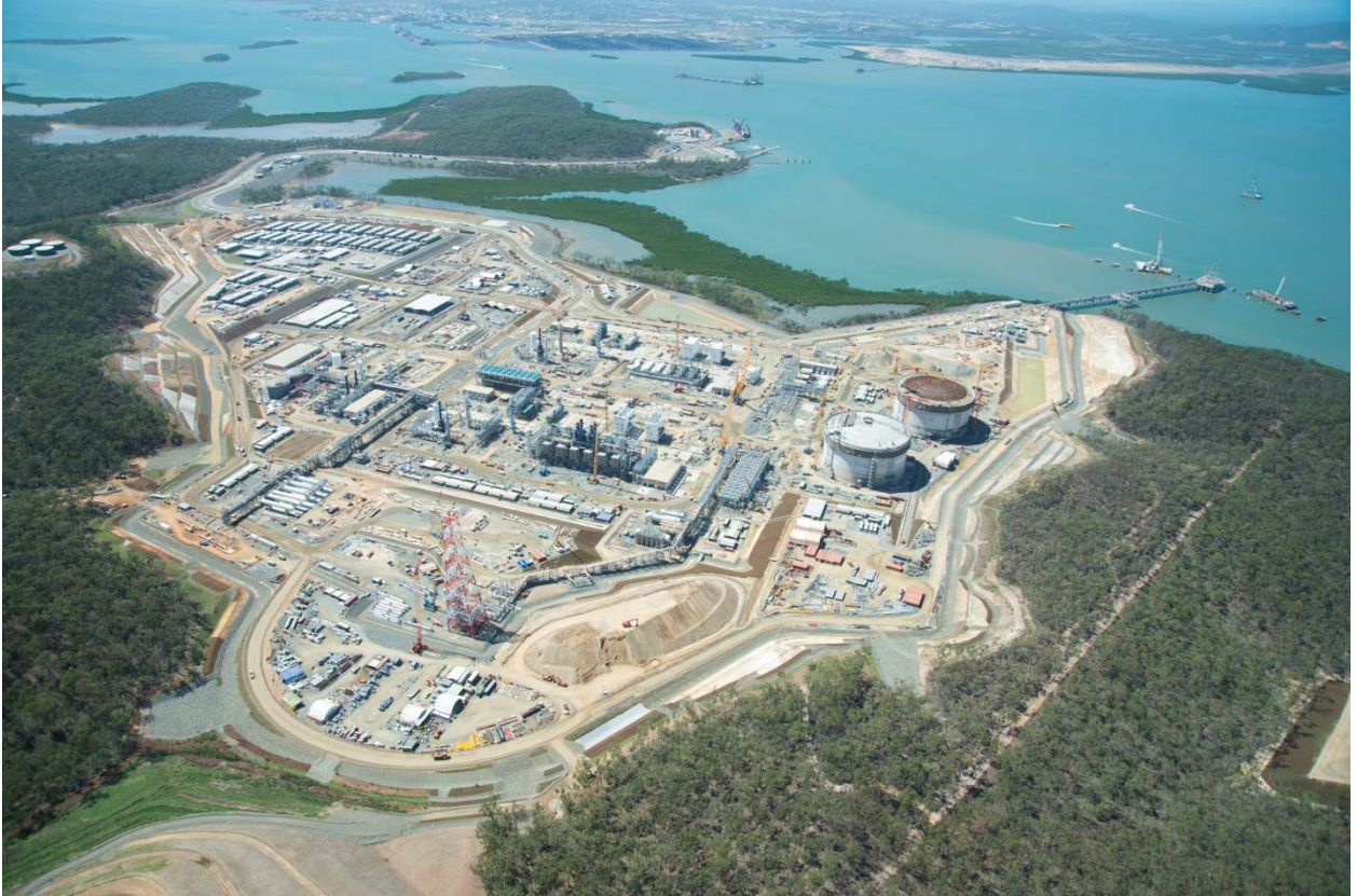
GLNG plant site on Curtis Island, 2 December 2013.
