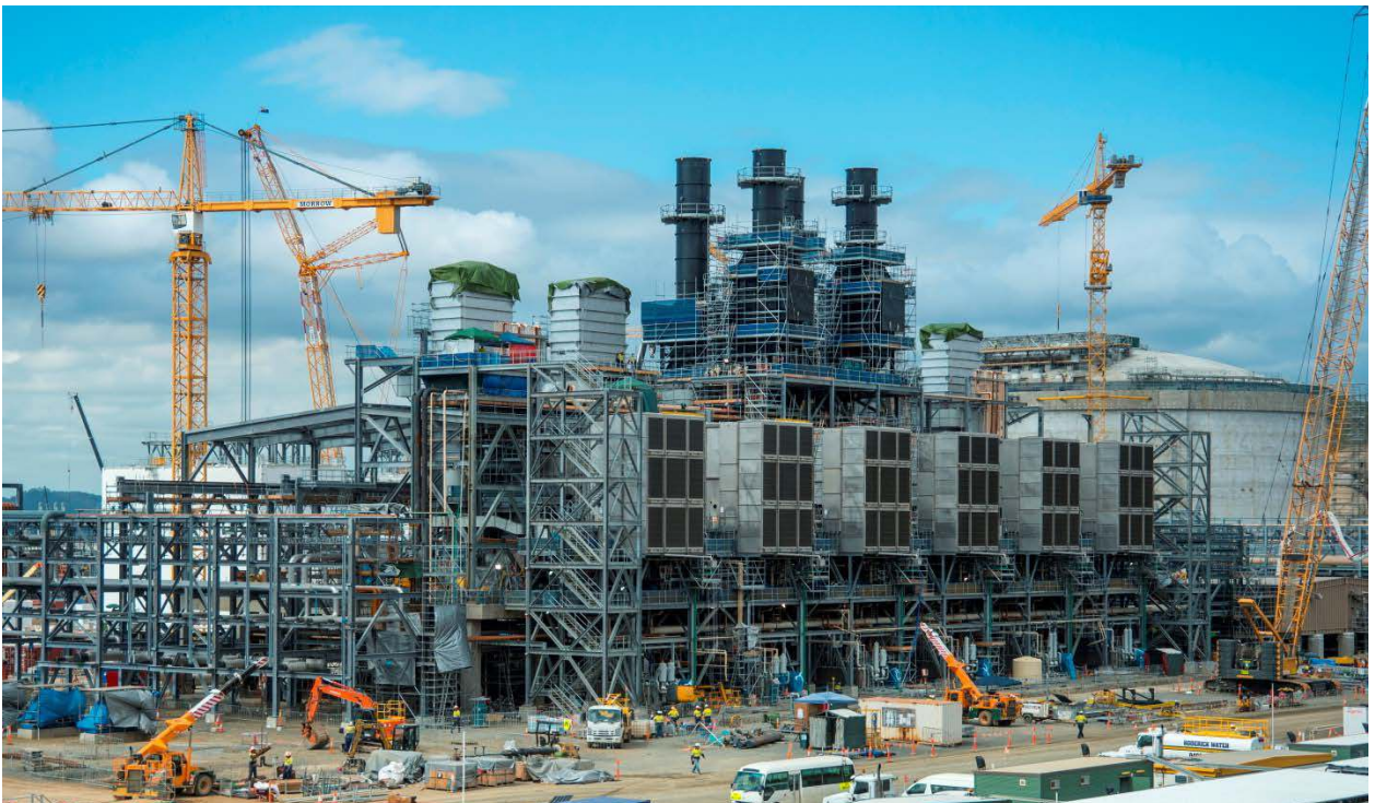
Train 1 compressor deck on Curtis Island with LNG tank B in the background, 2 December 2013.
