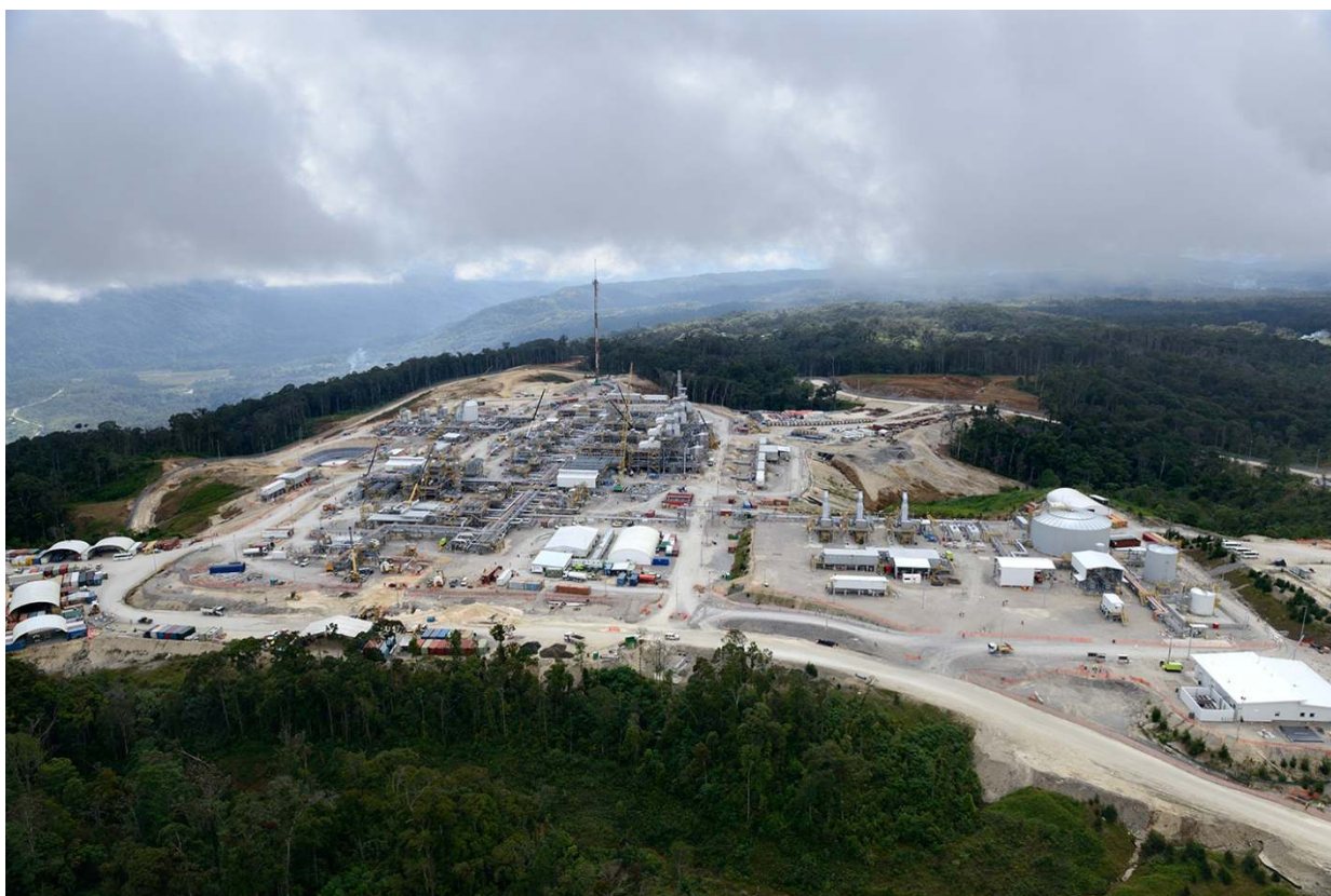
Hides Gas Conditioning Plant, PNG LNG, November 2013.
