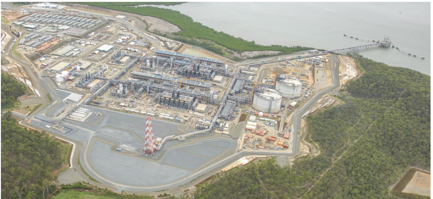
GLNG, Curtis Island, January 2015.
