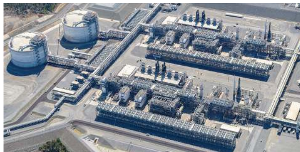
GLNG Train 2 started producing liquefied natural gas (LNG) on 26 May 2016.
