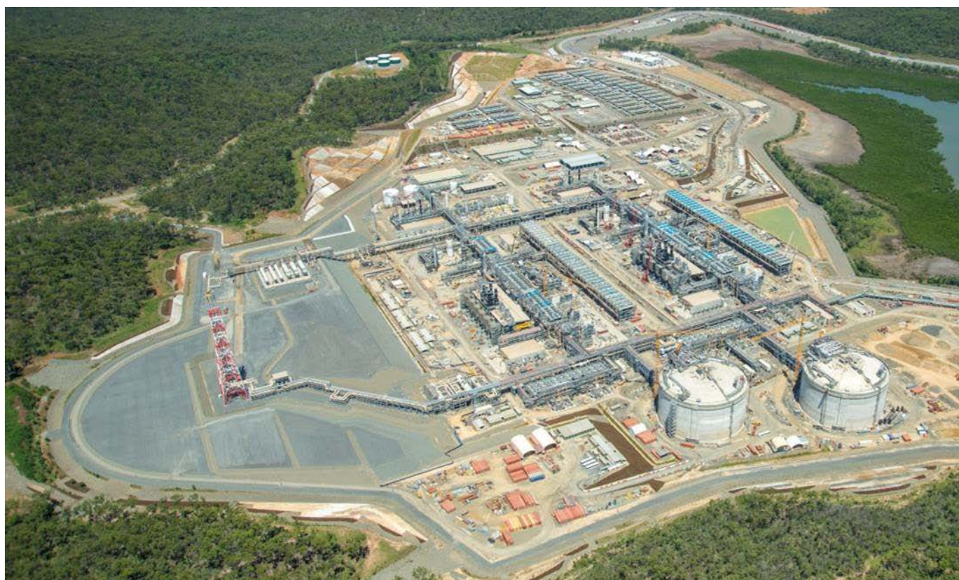
GLNG plant, Curtis Island, February 2015
