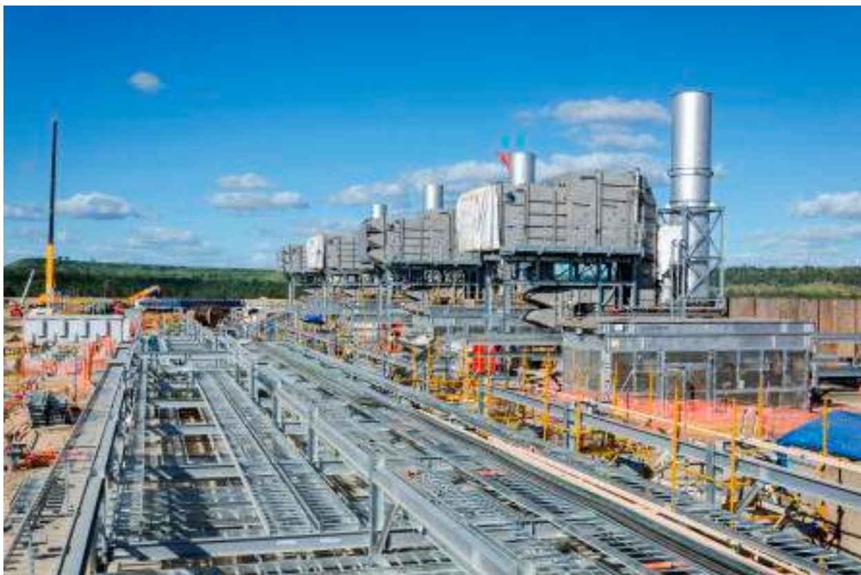
Fairview Hub-4 compressor station construction, March 2013
