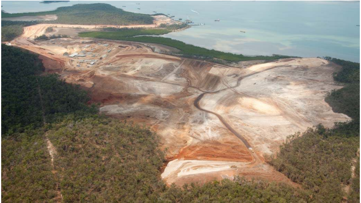
Aerial view of the cleared GLNG site on Curtis Island, 5 October 2011.
