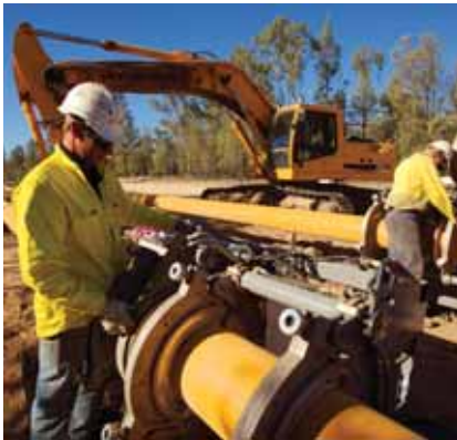
Pipelaying operations, Fairview coal seam gas field.
