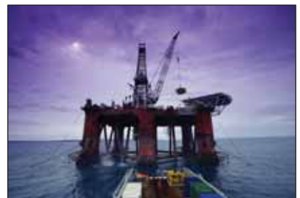
Henry and Kipper gas projects sanctioned, part of Santos' next wave of development projects.
