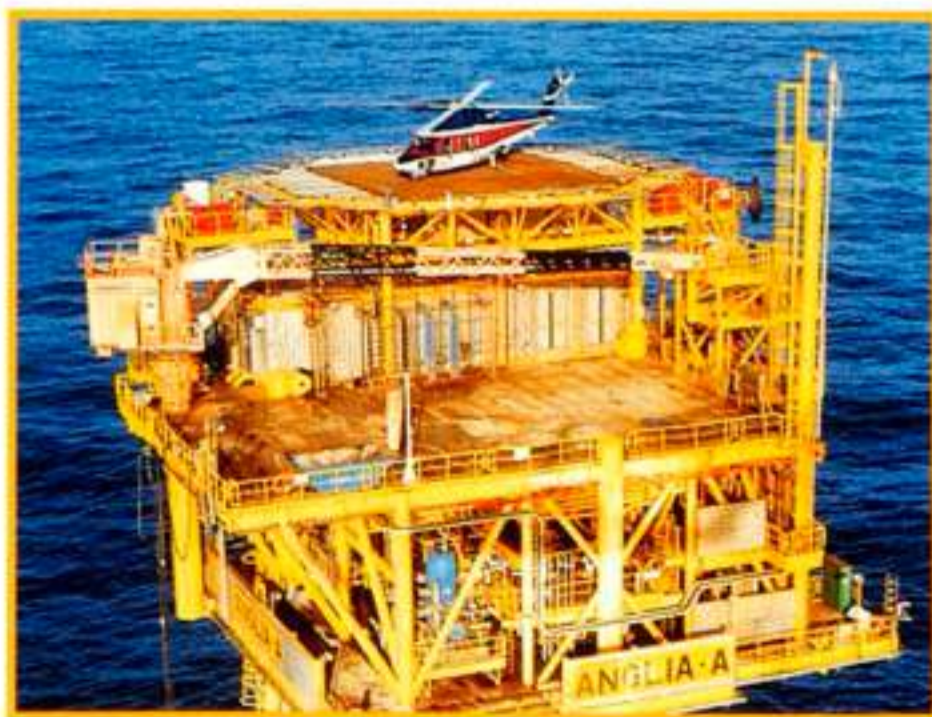
Above Anglia, North Sea, United Kingdom. Helicopter landing on production facility - Anglia field.
