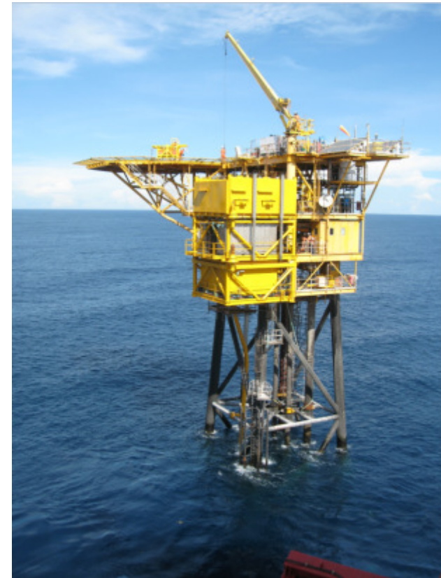
John Brookes platform with Spar wing deck module
