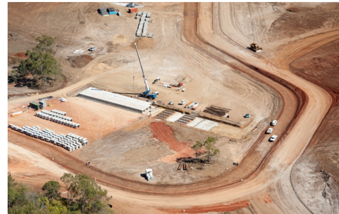
Culvert installation, Curtis Island
