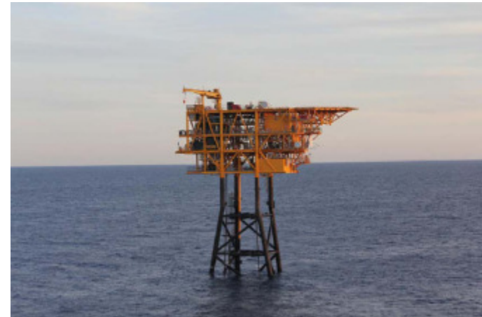
Reindeer wellhead platform
