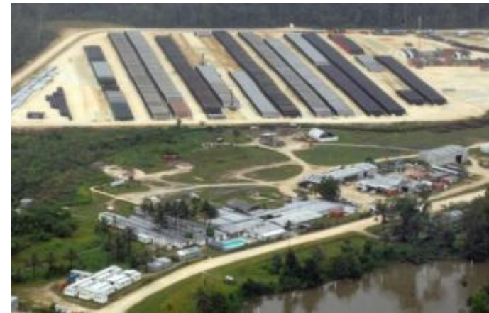
Line-pipe at Kopi shore base
