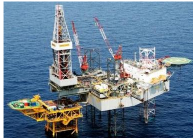
Chim Sáo wellhead platform and drilling rig
