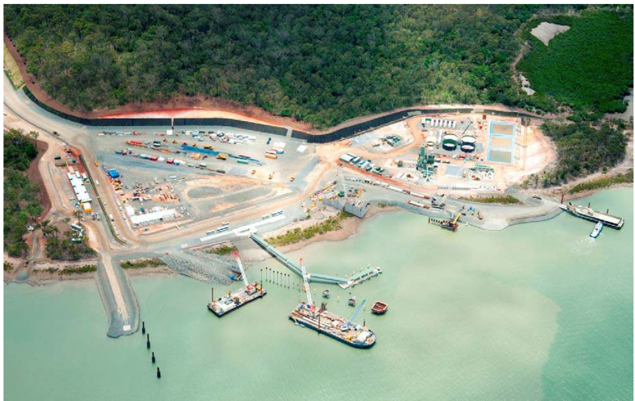
Aerial view of the GLNG material offloading facility site on Curtis Island, 3 January 2012.
