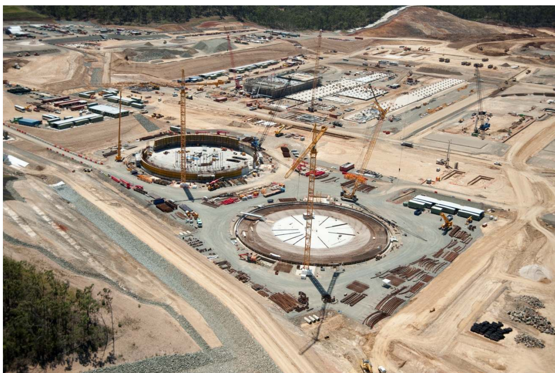
Above: LNG tanks with trains 1 and 2 construction in the background, October 2012.
