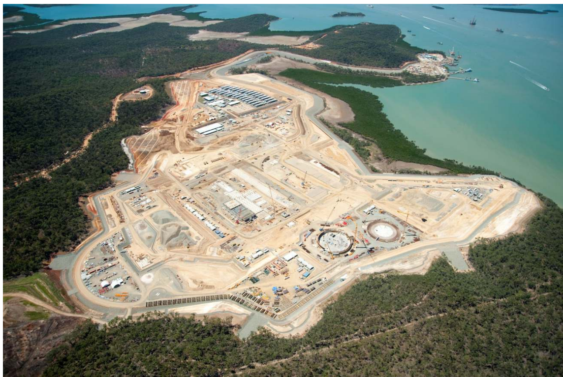
Above: GLNG plant site, October 2012.
