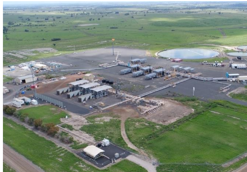
Scotia production facility - after
