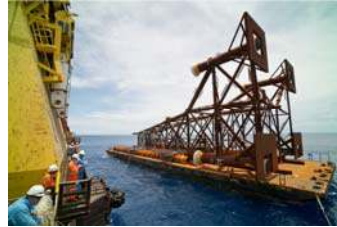
Reindeer jacket ready for installation
