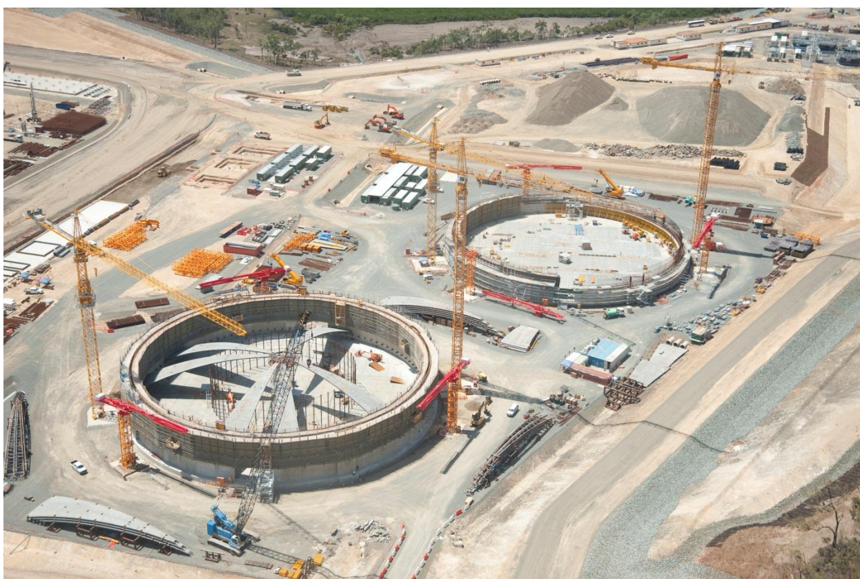
LNG tank construction, 4 January 2013
