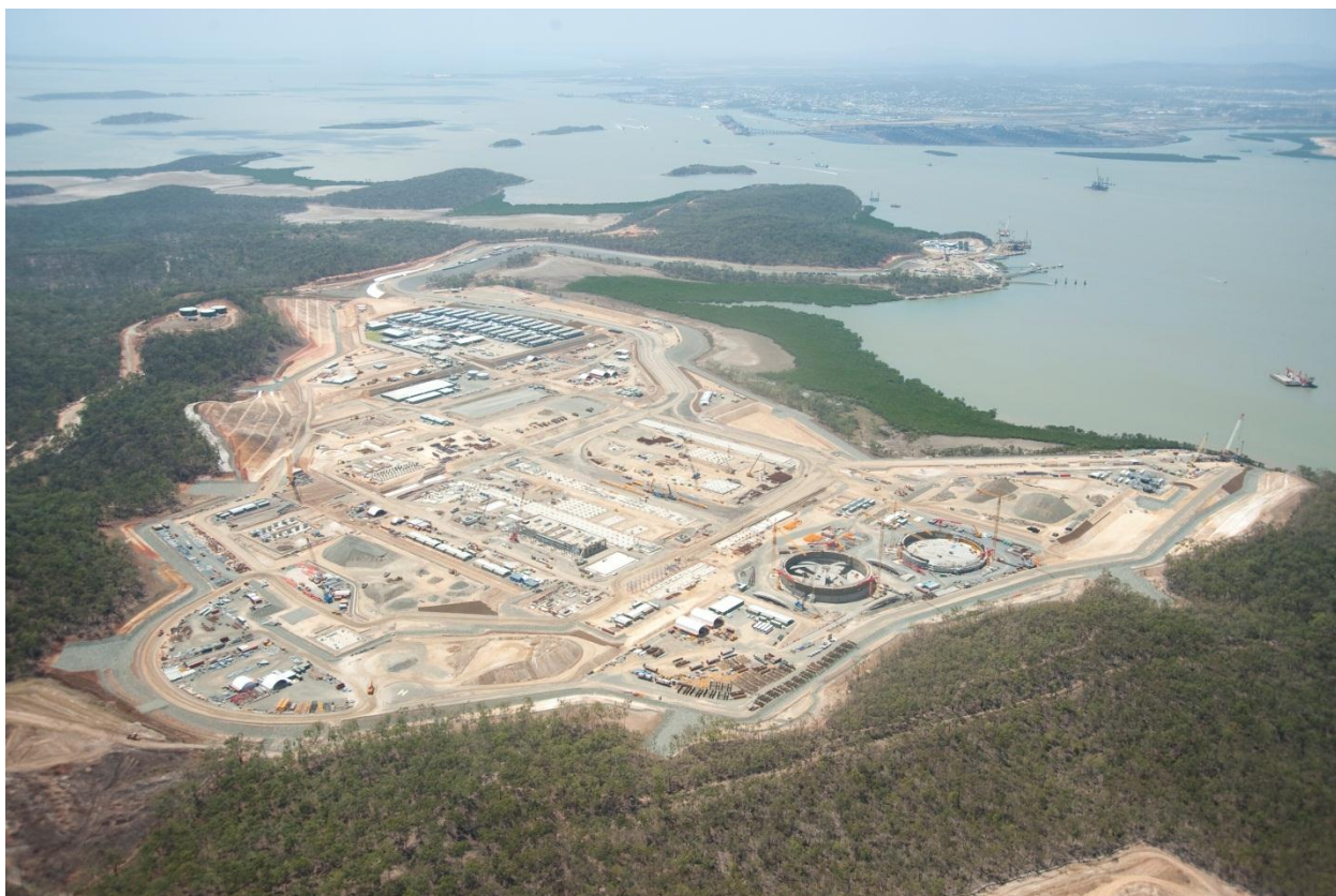
GLNG plant site, 4 January 2013.
