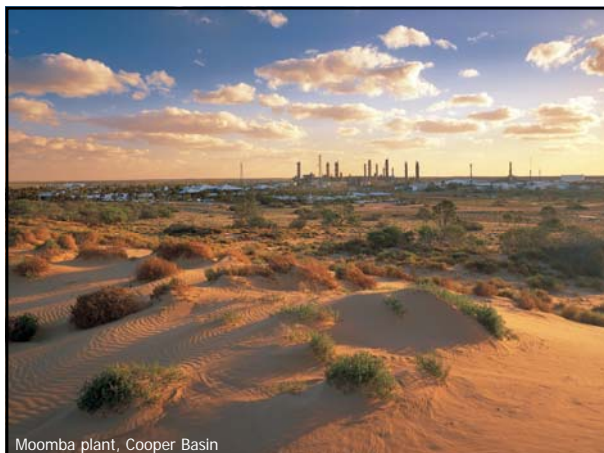
Moomba plant, Cooper Basin
