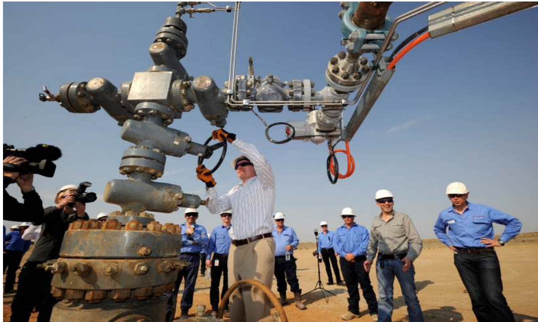
Moomba 191: SA Premier Jay Weatherill opens Australia's first producing shale well
