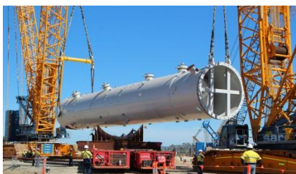
Train 2 carbon dioxide absorber rising in to position – click here for high res image
