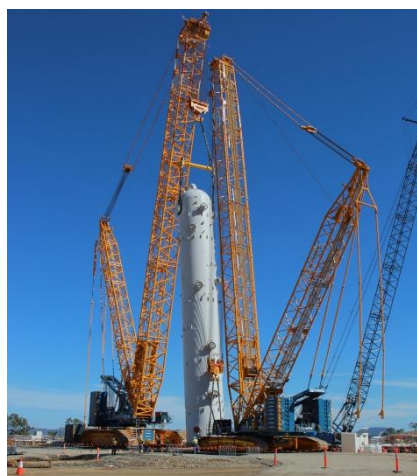
Train 2 carbon dioxide absorber rising in to position – click here for high res image
