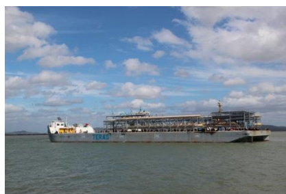
First prefabricated steel modules arriving from Batangas, Philippines – click here for high res image
