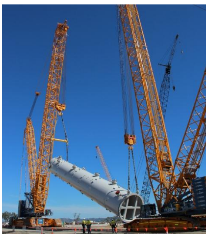
Train 2 carbon dioxide absorber rising in to position – click here for high res image
