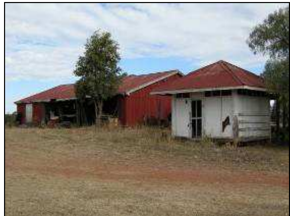
Figure 4.65: Shed and disused meat locker (Image: ARCHAEO 2008).
