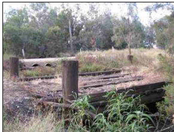
Figure 4.95: Wooden road bridge with current concrete bridge in background (Image: ARCHAEO 2008).
