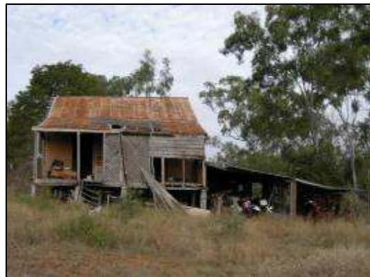
Figure 4.18: Former Workers' Cottage (Image: ARCHAEO 2008).
