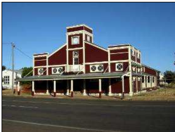
Figure 4.1: Warroo Shire Hall. The hall is currently being repaired as can be seen by the fencing and new external paint (Image: ARCHAEO 2008).
