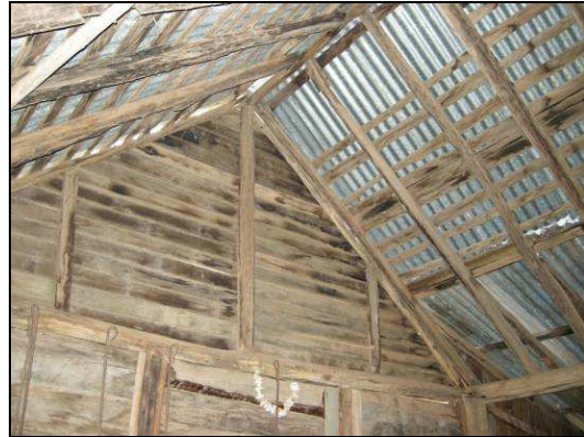
Figure 3.11: Roof structure of stables, (Image: ARCHAEO 2008).
