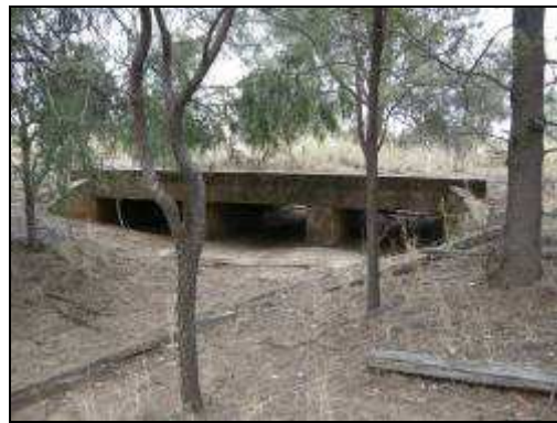
Figure 4.39: Concrete bridge (Image: ARCHAEO 2008).
