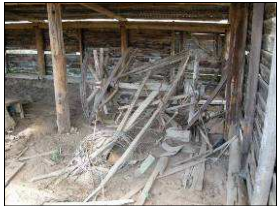
Figure 4.61: The remains of the dray within the machinery shed (Image: ARCHAEO 2008).
