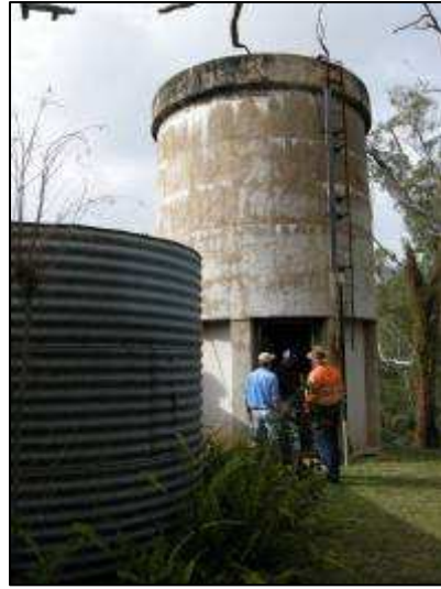
Figure 4.20: Concrete water tank (Image: ARCHAEO 2008).
