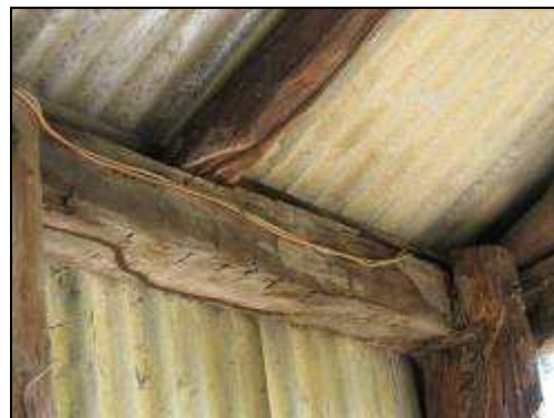
Figure 4.97: Hand blazed timbers within the older cottage (Image ARCHAEO 2008).
