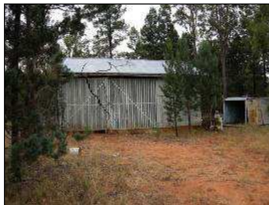
Figure 4.103: Main shed with generator building to the right (Image: ARCHAEO 2008).
