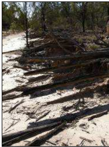
Figure 4.32: Part of the Corduroy Rd near Surat showing the water damage from the borrow pit overflow (Image: ARCHAEO 2008).
