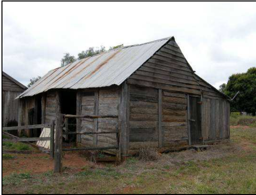
Figure 3.10: Timber slab stables (Image: ARCHAEO 2008).
