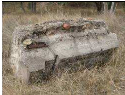
Figure 4.123: Excavated concrete engine bed (Image: ARCHAEO 2008).
