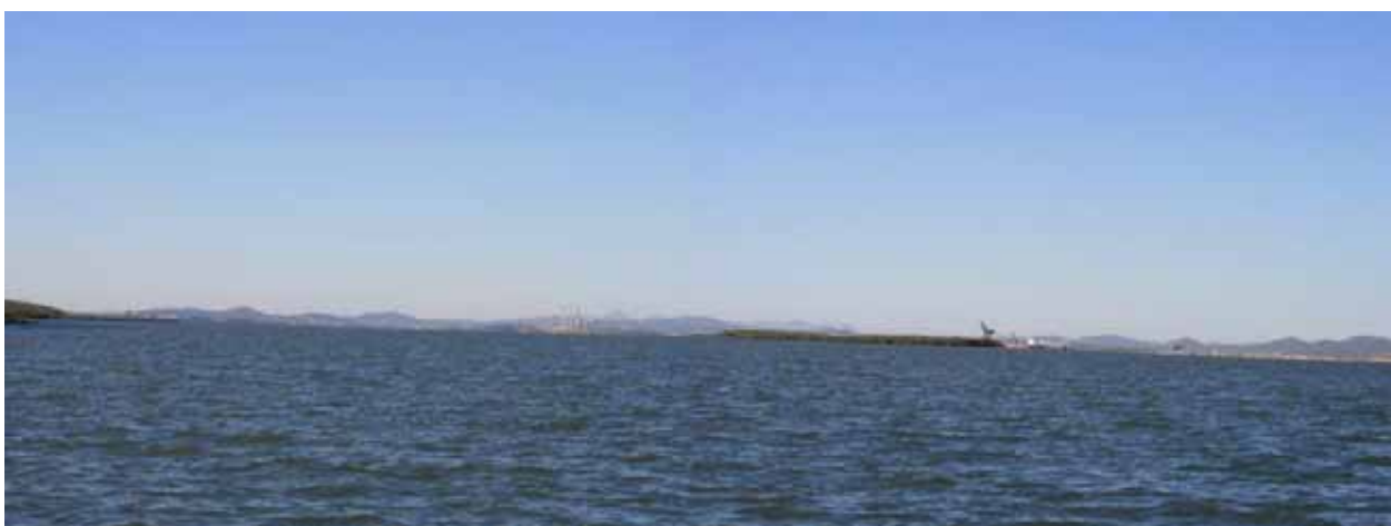
VS 24 - The Narrows shipping channel, view to south east
