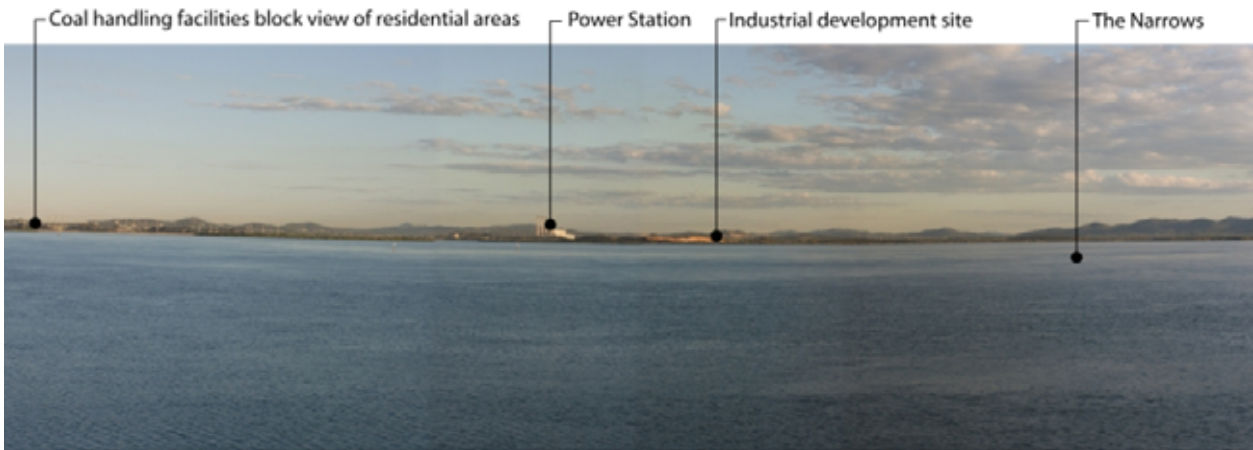
Location 5 - View south towards Gladstone Power Station
