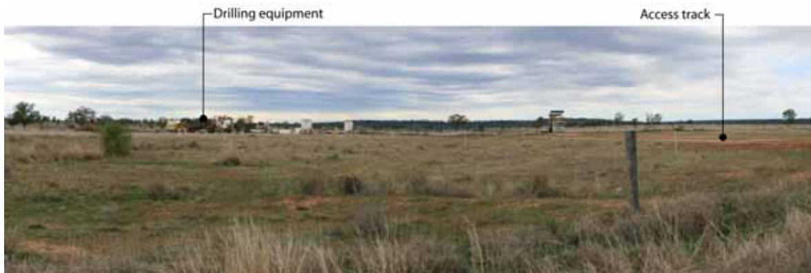
Plate 16 Typical exploration drilling operations viewed from a public road
