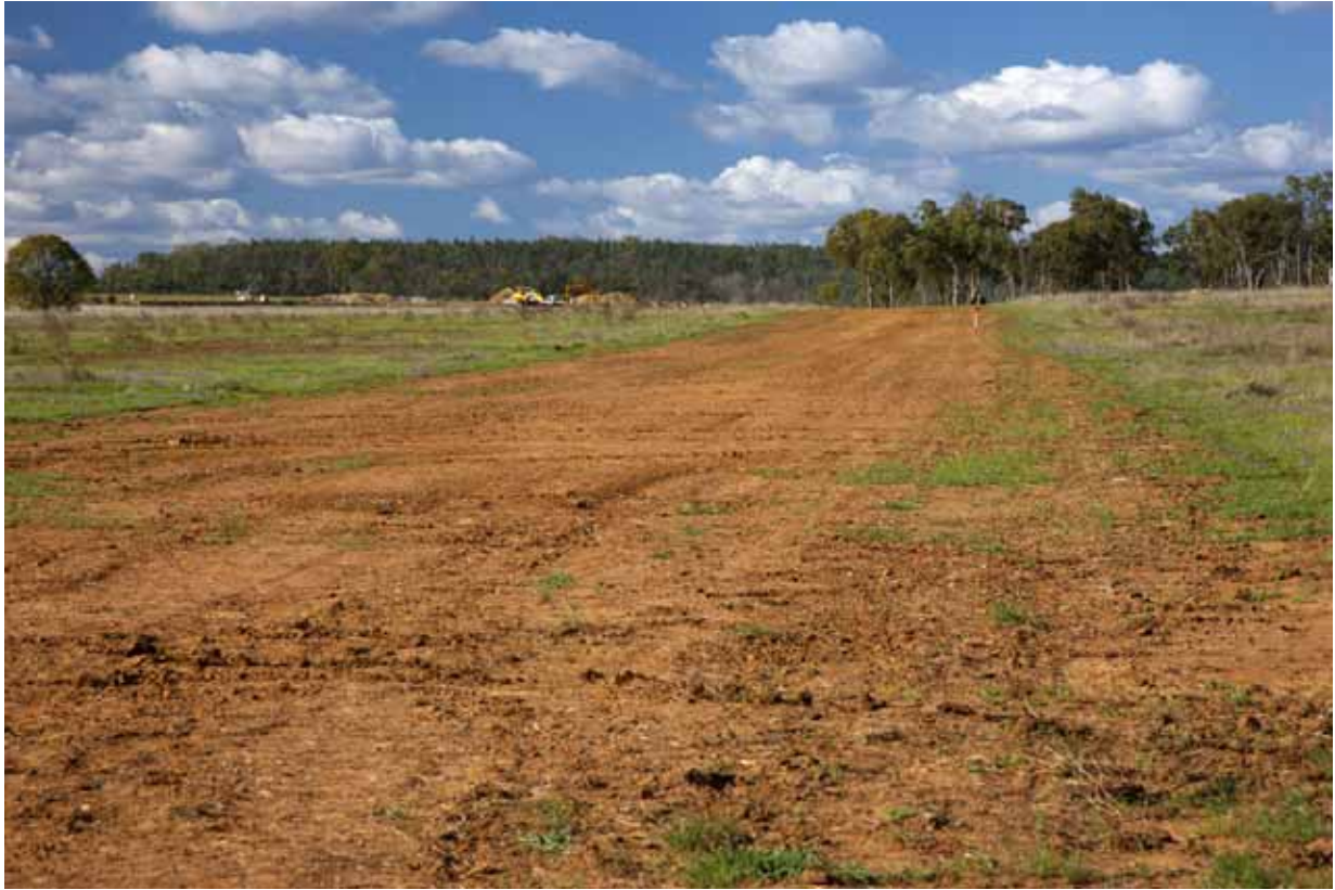
Plate 41 Typical pipeline easement after backfilling trench and prior to revegetation works
