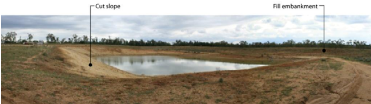
Plate 29 Water storage dam constructed near Coxon Creek
