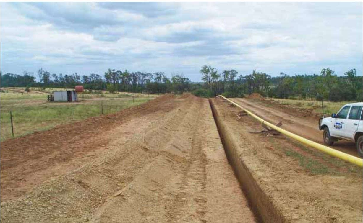
Plate 40 Typical trench with 'pipe string' laid out ready for installation
