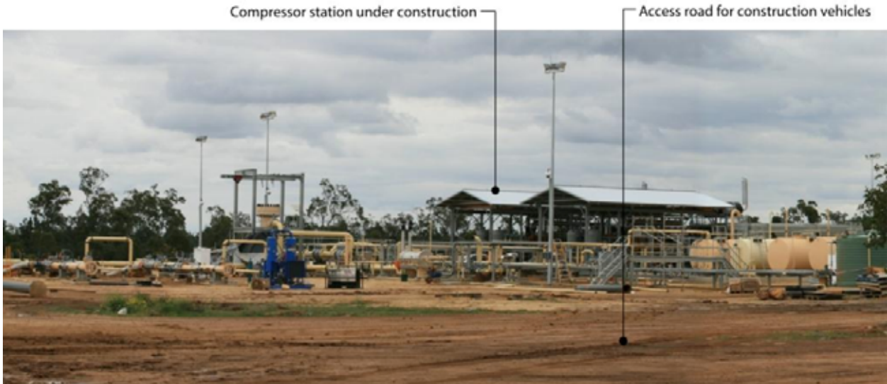
Plate 32 Fairview compressor station under construction near Springwater Camp
