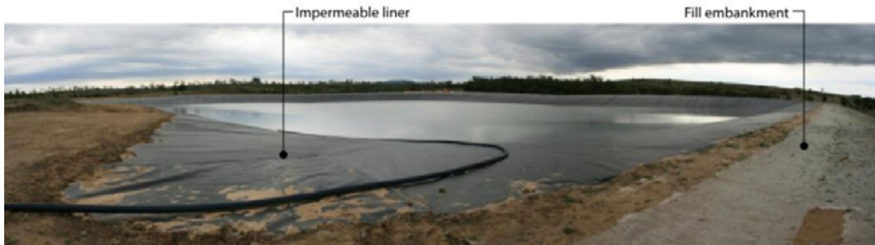
Plate 30 Water storage dam constructed with impermeable liner
