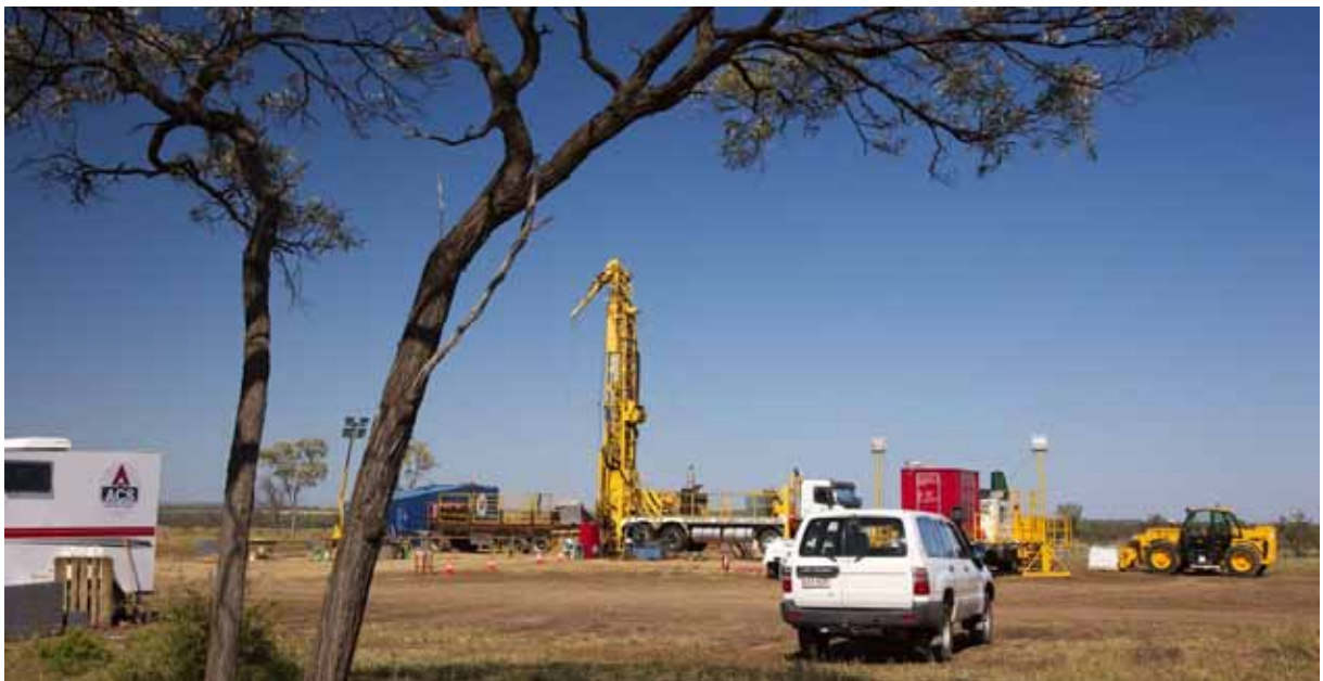
Plate 18 Exploration drilling rig
