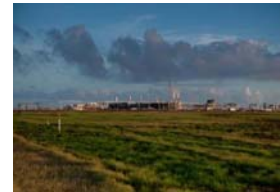
Devil Creek gas plant
