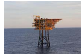
Reindeer wellhead platform installed
