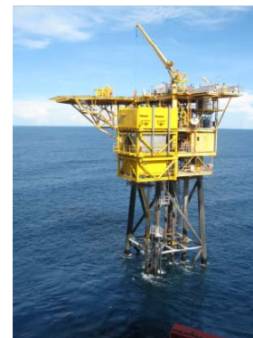
Wing deck module installed on John Brookes platform
