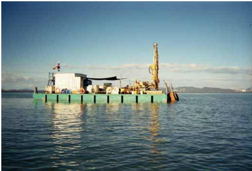
Plate 1: Looking east across the Targinie Channel
