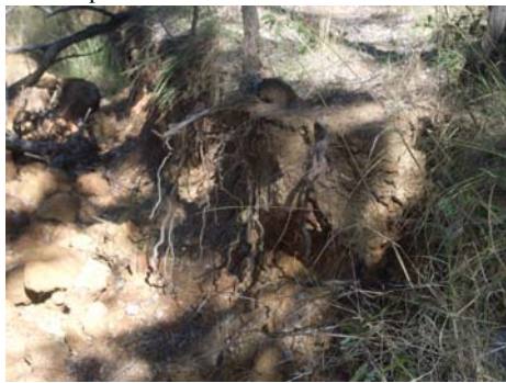
Photo: Eroded Downstream Bank
