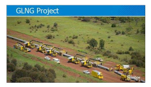
Construction of the pipeline is also progressing. Around 220 kilometres has been cleared and graded, 180 kilometres of pipe strung and over 11,000 welds completed.
