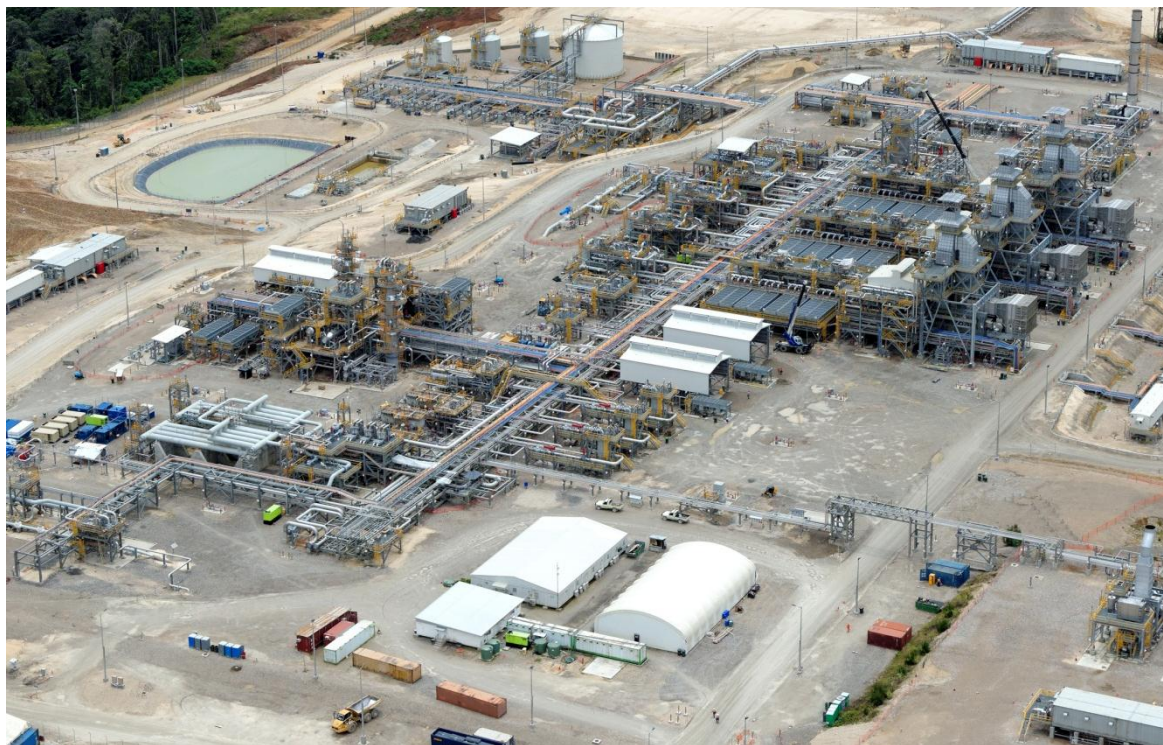
Hides Gas Conditioning Plant
