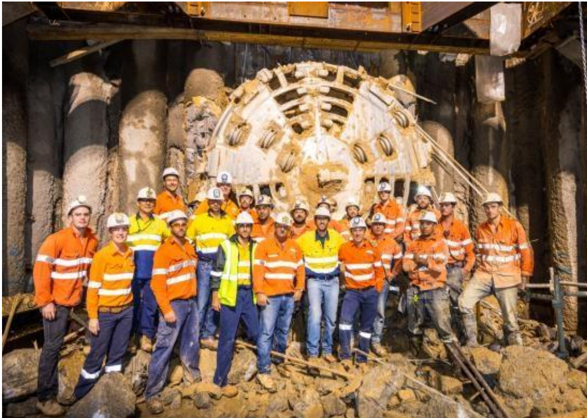
Marine crossing tunnel break-through on 3 February 2014
