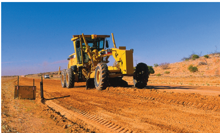
Roadwork activities can be a source of noise.
