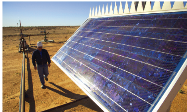
Inspection of solar powered air compressor, Cooper Basin.
