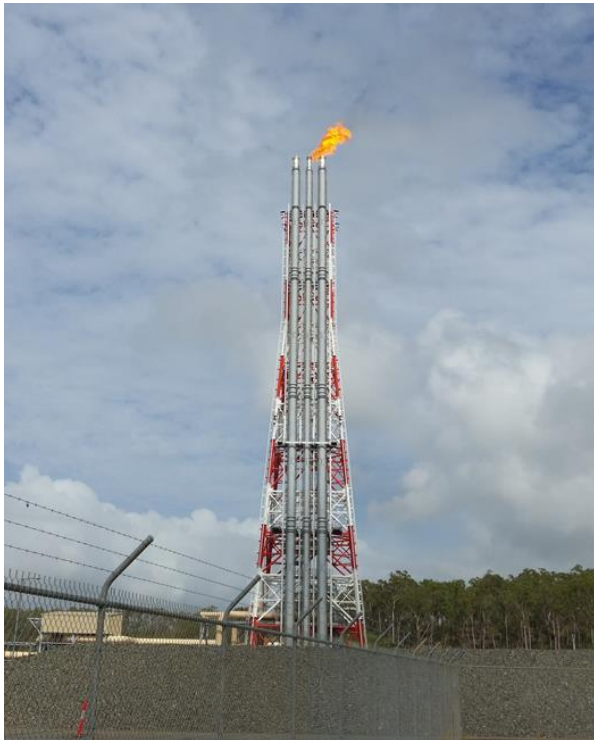
GLNG flare stack, Curtis Island, March 2015
