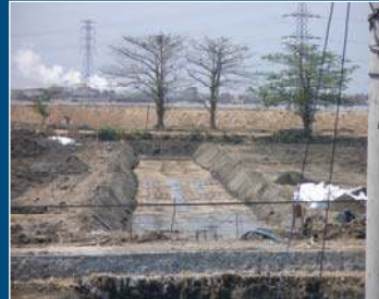
Spillway construction
