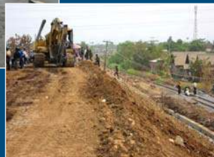
Levee to protect railroad
