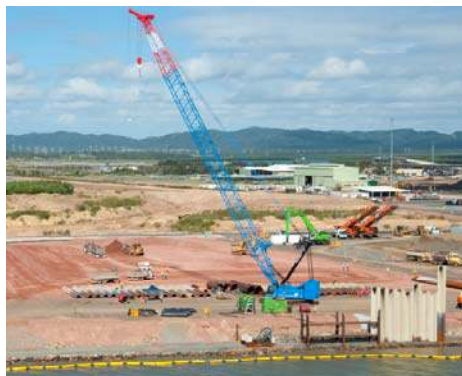
Early construction works at GLNG logistics facility, Gladstone harbour
