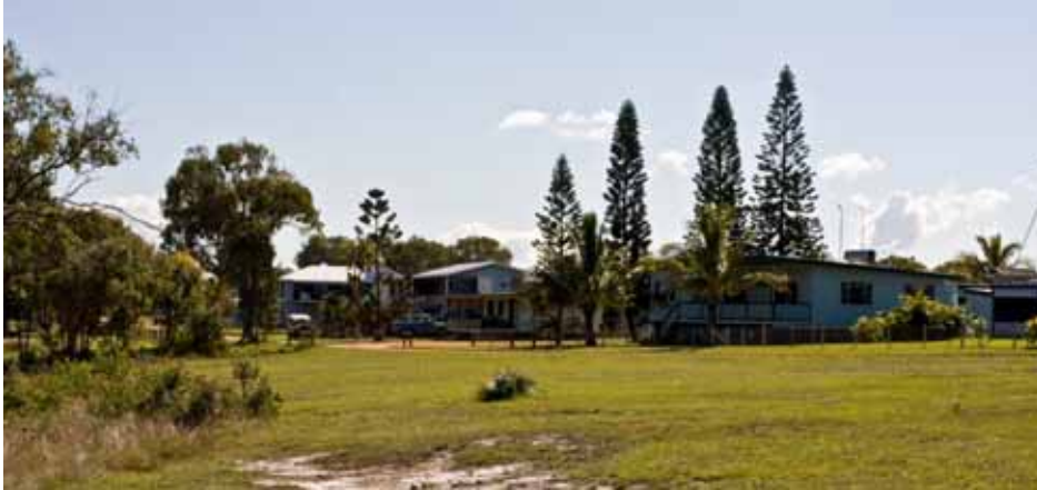
Plate 8.12.4 LCZ 4 - South End Township and Jetty
