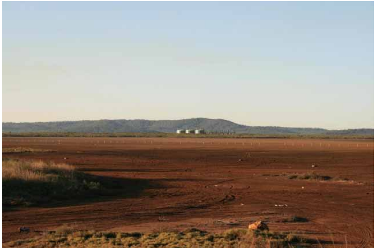
Plate 8.12.22 Visual Simulation 5a - View from Mount Larcom to Gladstone Road at Reid Road intersection, with the LNG facility visible on Curtis Island (white LNG storage tanks in centre of photo, flare stack above right hand tank, LNG train to right of tanks)
