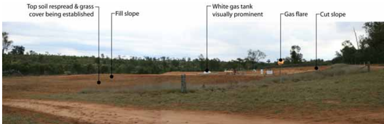
Plate 6.12.20 Production Well Lease on Undulating Landform Showing Cut and Fill Slopes Prior to Revegetation
