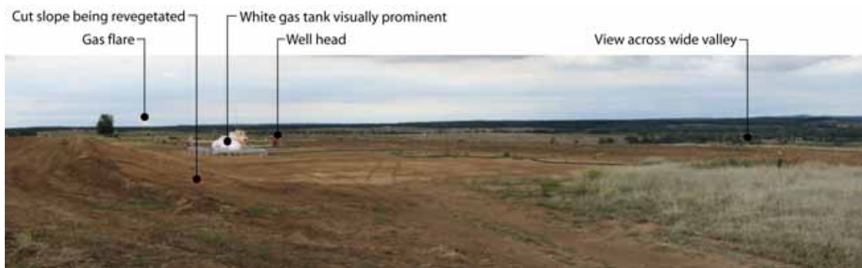
Plate 6.12.22 Production Well on Ridge Top with Cut and Fill Slopes Prior to Revegetation
