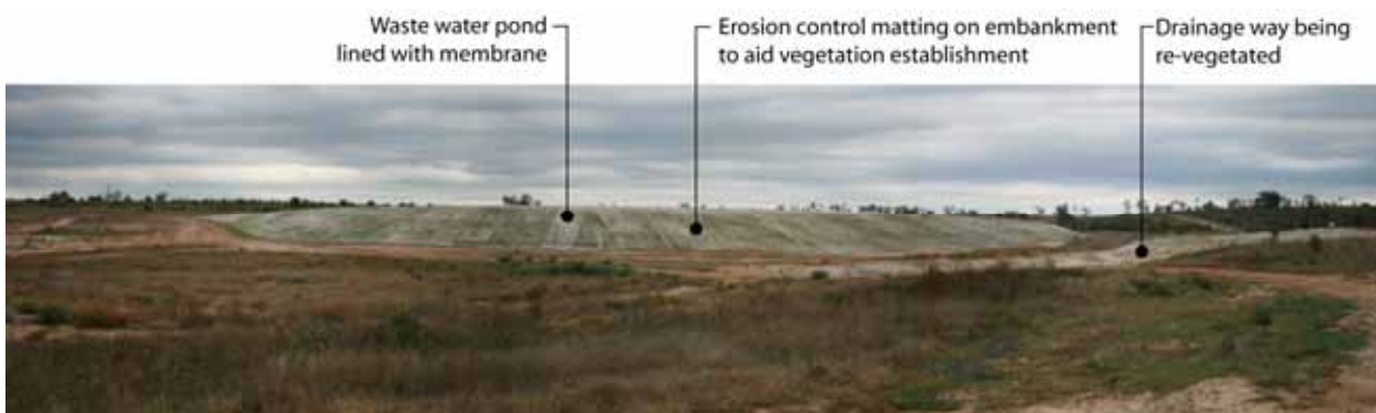
Plate 6.12.30 Water Management Pond Embankment with Erosion Control Matting used to Establish a Protective Grass Cover
