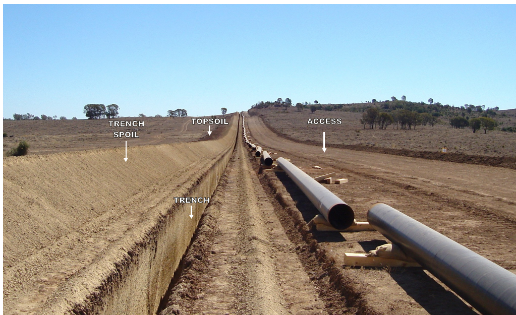
Figure 3.7.2 Cleared Pipeline ROW
