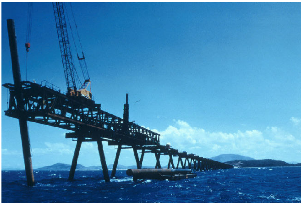
Figure 3.8.1 "Hand Over Hand" Construction Method
