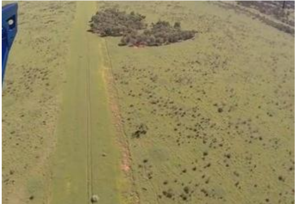
Aerial view of the reinstated pipeline route in the Arcadia Valley
