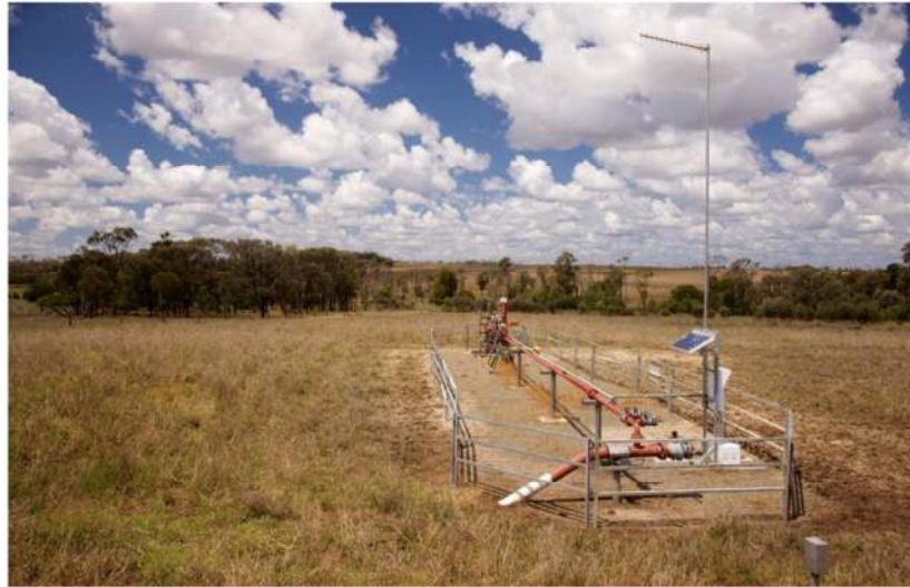
Production well at Scotia, Queensland
