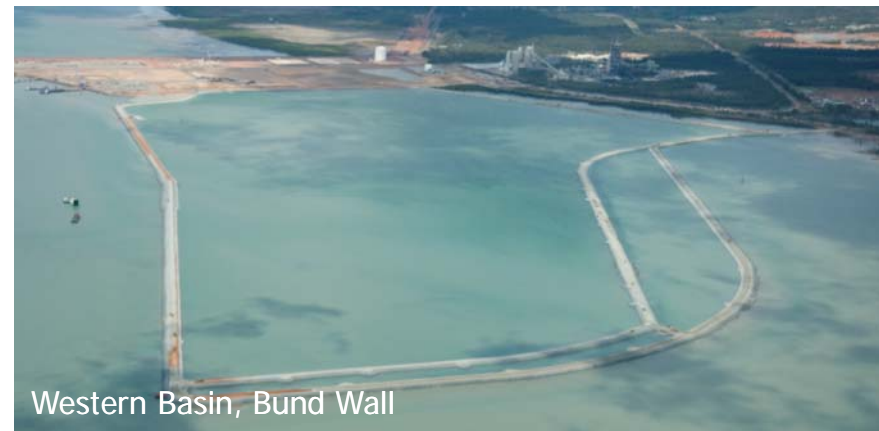
Dredging, Gladstone Harbour
